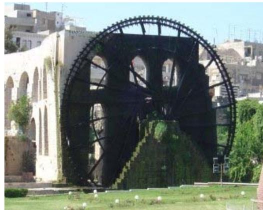
*Al-Mohammediyah: the biggest and oldest Noria in the world. A superb example of a simple technology totally self sufficient in energy, that has raised water for over a thousand years.*
