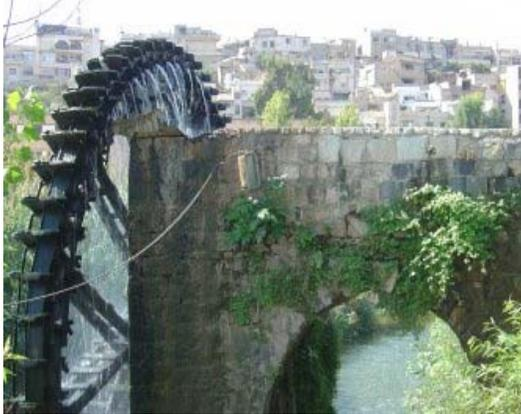
*Details of a self operated waterwheel of 8 m diameter, Hama, 2005*
